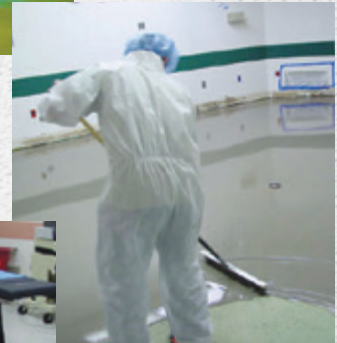
Arroyo Grande Regional Hospital Arroyo Grande, CA Quirófanos
