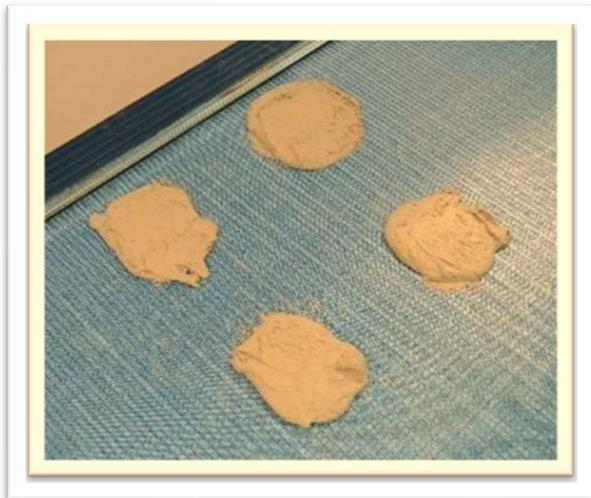
Mix ARDEX mortar in accordance with its technical data sheet.
