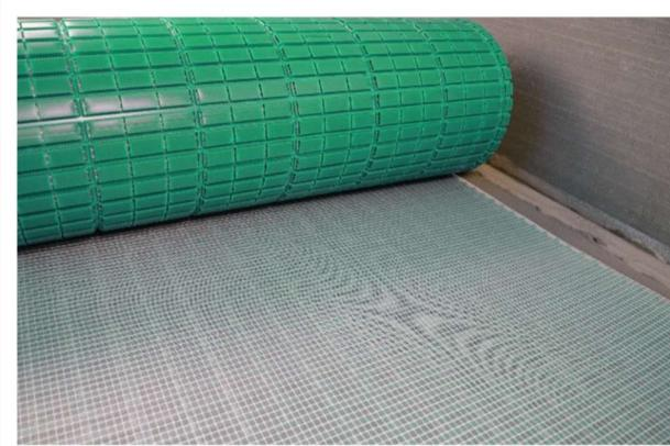
Roll the mat into place and cut to size using ARDEX FLEXBONE Shears or a utility knife. Ensure that the waterproofing or vapor retarder membrane is not cut.
