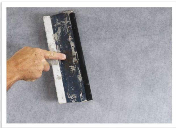
Install ARDEX TLT Membrane as a Vapor Retarder\* with an ARDEX Mortar over the sloped substrate and place up to the plastic side of the ARDEX US 422 ProDrain Tape, covering the fleece. Please refer to the ARDEX TLT technical data sheet for application information.
