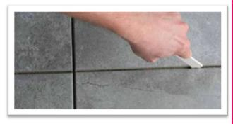
NOTE: For tile larger than 16"x16" (40 cm x 40 cm) and/or pattern installations, use ARDEX SX 100% Silicone Sealant in place of grout.
