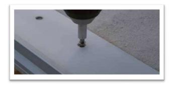
Cut and install the appropriate size ProFin Profile and the inside and outside ProFin corners on the perimeter of the area of installation. Place galvanized fasteners in every other hole or as necessary to secure the profiles.
