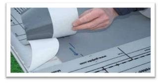
Install the ARDEX US 420 ProDrain Tape along the inside edge of the ProFin Profile. Ensure that the tape covers all fasteners. The dotted line on the tape should be in alignment with the inside edge of the ProFin Profile.
