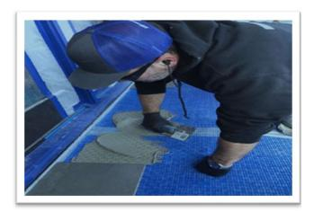
Installation should proceed in accordance with ANSI A 108.5. After mixing, apply the mortar directly over the mat with the flat side of a notched trowel (keying in) to obtain a solid mechanical bond.
