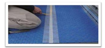
Align and join the membrane sheets using the self-adhesive ARDEX UD 158 Seam Reinforcement Mesh Strip.
