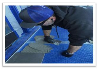
Installation should proceed in accordance with ANSI A 108.5. After mixing, apply the mortar directly over the mat with the flat side of a notched trowel (keying in) to obtain a solid mechanical bond.
