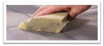
NOTE: Grouting must NOT be applied around the perimeter edge. All installations must include soft joints using ARDEX SX™ 100% Silicone Sealant in accordance with ANSI A 108.01-3.7 and TCNA EJ 171.
