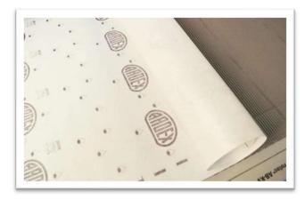
Install ARDEX SK 175™ Membrane as a Vapor Retarder\* with an ARDEX Mortar over the sloped substrate and place up to the plastic side of the ARDEX US 420 ProDrain® Tape, covering the fleece. Please refer to the ARDEX SK 175 technical data sheet for application information.
