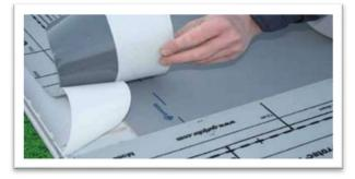
Install the ARDEX US 420 ProDrain Tape along the inside edge of the ProFin Profile. Ensure that the tape covers all fasteners. The dotted line on the tape should be in alignment with the inside edge of the ProFin Profile.
