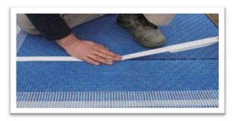
Spacing between the mat sheets honoring movement and transition joints should be covered with tape to protect against the entry of mortar and grout to the substrate below to avoid bonding the mat to the substrate.
