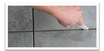
Allow ARDEX X 90 to dry for 2 hours (70°F / 21°C), then clean the grout joints of any excess mortar. Also, clean the tile or stone surface and allow to dry. Once the surface is dry, mix and apply ARDEX FL™ Rapid Set Sanded Grout or ARDEX WA™ Epoxy Grout in accordance with the corresponding technical data sheet, and place into the grout joints.
