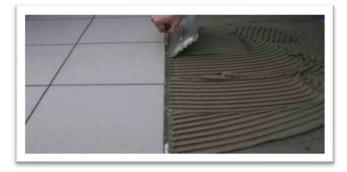
Apply ARDEX X  $90^{\text{TM}}$  OUTDOOR to the back of the tile or stone using a flat trowel and then install the tile.
