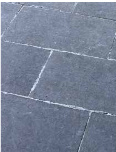
EFFLORESCENCE
