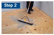
Sweep or vacuum debris from the substrate. In intermittent wet areas or where waterproofing is required, moisture-sensitive substrates, such as gypsum, must be protected from water damage by priming with ARDEX P 51 and installing ARDEX 8+9.
