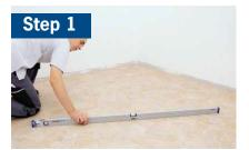
Check the substrate for load-bearing qualities, evenness and structural soundness. If leveling is necessary, a product such as ARDEX Liquid BackerBoard may be used.
