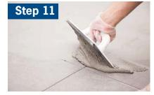
Due to properties of plastic membranes, mortar type, tile type, tile size and climactic conditions, the mortar curing time required prior to grouting may vary. ARDEX mortars allowable for use with ARDEX uncoupling membranes typically permit grouting in 3 - 24 hours.
