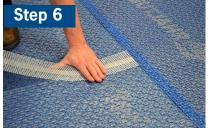
Use the self-adhesive ARDEX UD 158 Seam Reinforcement Mesh Strip to bond seams at the ends and cut areas of the membrane where there is no overlapping self-adhesive mesh.
