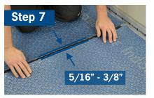
Leave a joint minimum width of 5/16" - 3/8" (8 - 10 mm) for expansion and field perimeter joints that sub-divide large areas, doorways, etc.
