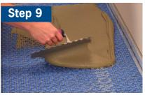
Using the flat side of a trowel, fill and smooth ARDEX UI 720 FLEXBONE with the appropriate ARDEX mortar so that the mortar is flush with the top of the mesh.
