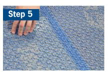
Butt joint the membrane sections with the protruding edges of the self-adhesive mesh weave. Overlap onto the adjacent membranes.
