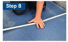
Cover the joints with self-adhesive ARDEX UD 156 Movement Joint Tape to protect against the entry of mortar and grout.
