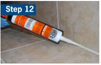
Fill movement and perimeter joints with an appropriate soft joint filler such as ARDEX CA 20 P or ARDEX SX.
