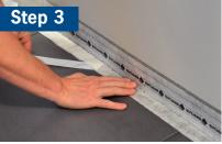
Along the perimeter walls and penetration of the covering, use ARDEX UD 146 Edge Insulation Strips with a self-sticking adhesive foot.
